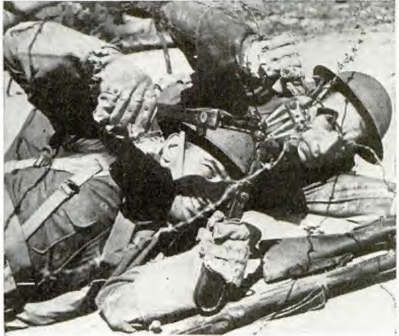
Big steel clippers bite their way through barbed wire as Army engineers clear a path for advancing troops. Note the heavy gloves and rifles within easy reach
